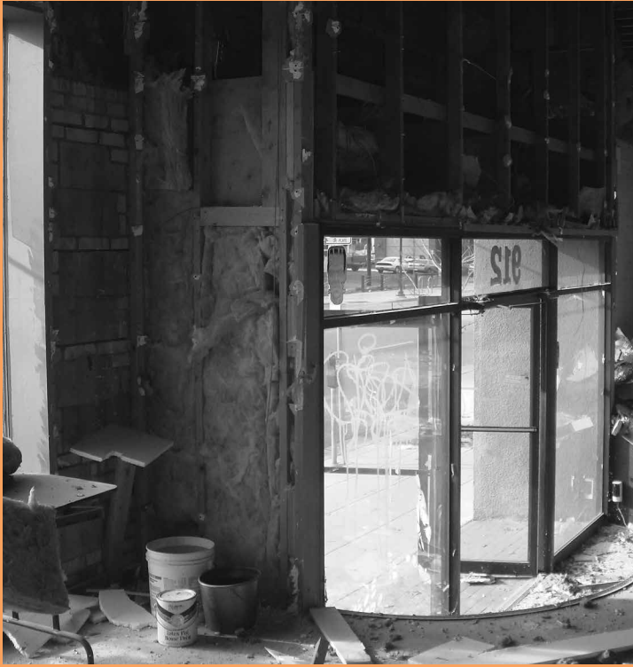
Looking back: Highpoint's front door before renovations.
